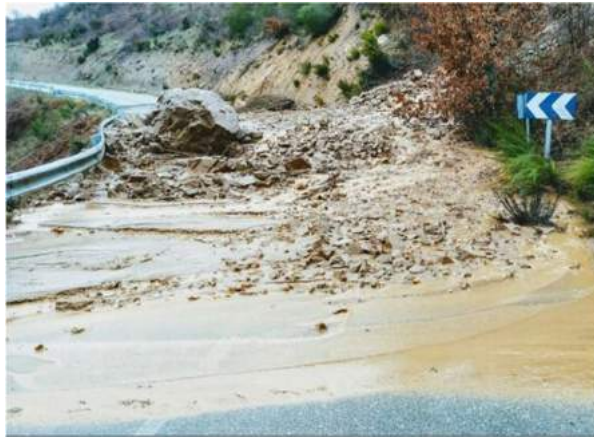
A landslide has cut the road that connects La Vida de Gordón with Villar del Puerto on 19 of December (province of León)
