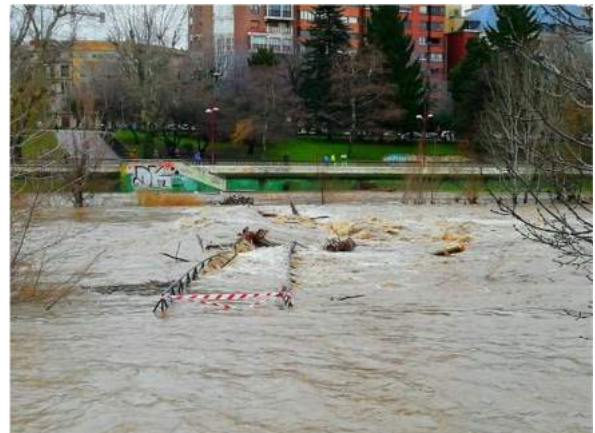
City of León, the gateway of La Condesa is again submerged and its structure completely damaged
