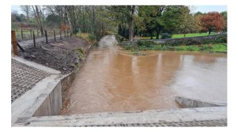
Figure 13: A view of the downstream side of the embankments at the St Vigeans FSA. River levels are controlled and well below the bank levels.
