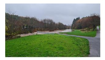
Figure 10: A view of operation 4 in The Dammy. This a low lying park area between Arbroath and St Vigeans where there is no river wall or deep bank and this area is a natural flood plain, so the design allows for water to lie here during flood events. Debris post
