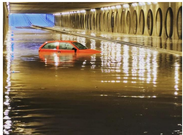
Figure 6: Flooded tunnel in Valencia, 03 May 2022. Credit: Policía Local Valencia
